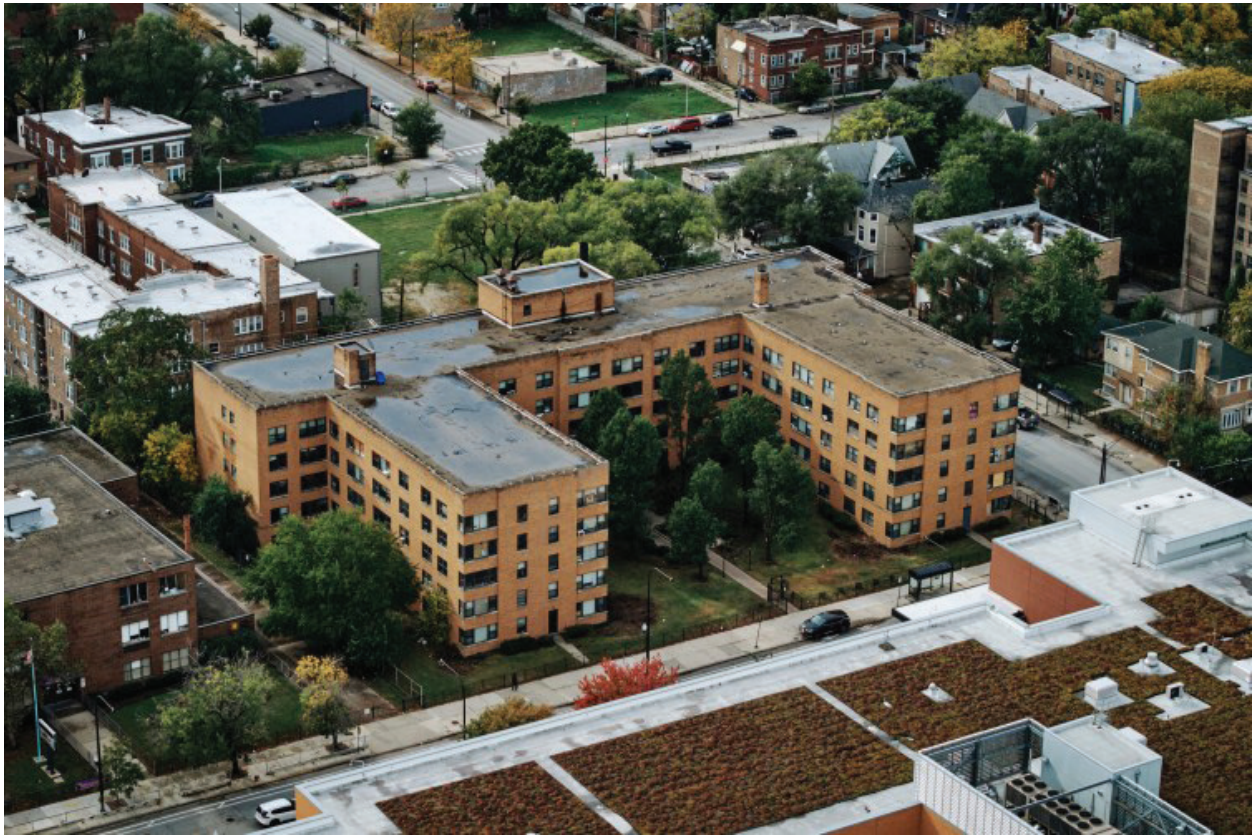
Image 8 An aerial view of the apartment building raided by federal agents in Chicago's South Shore neighborhood (Source: Mustafa Hussain for ProPublica) xxv
